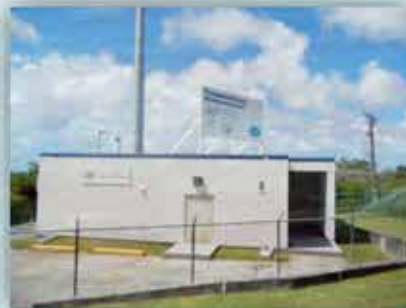
Pacific Telecom Inc. -Telecommunication facility in As Gonno, Saipan
