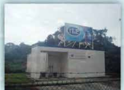
Pacific Telecom Inc. Telecommunication facility in Kagman, Saipan
